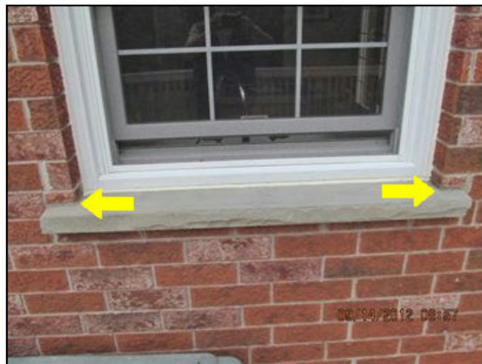
Caulk around window ledges
