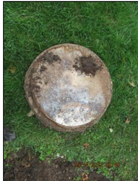
Outlet chamber lid showing deterioration
