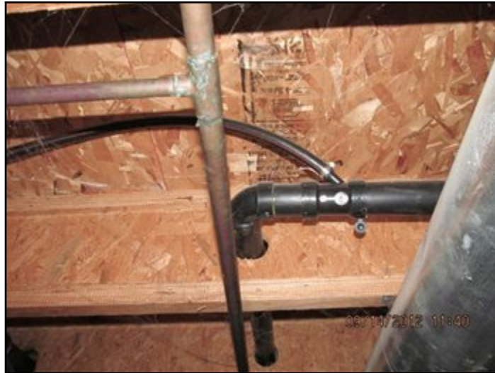
Existing water softener discharge location
