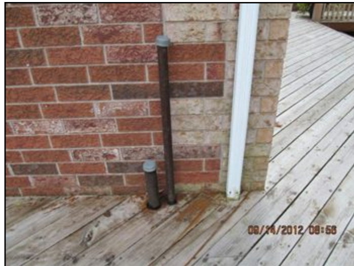
Location of oil fill and vent pipes
