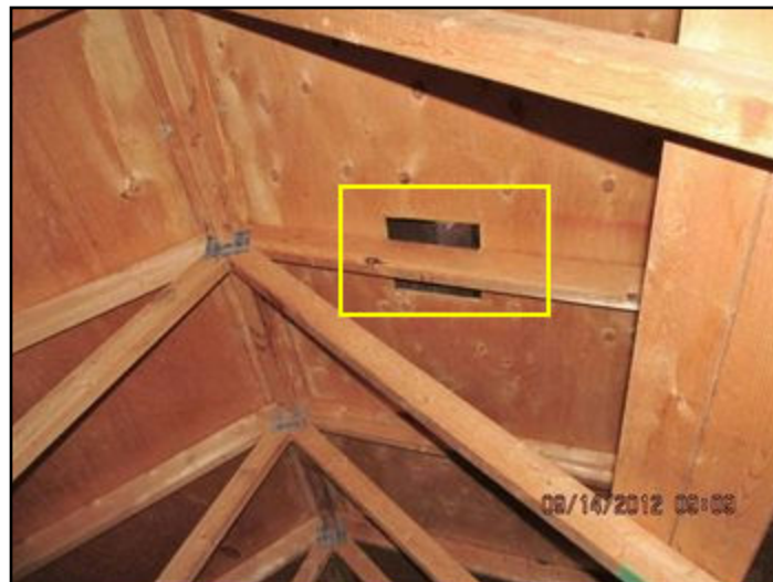
Roof vent not completely open
