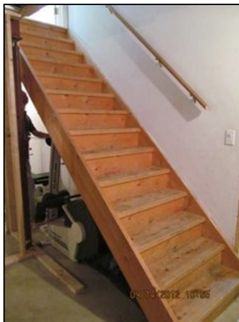
Guard rail missing
