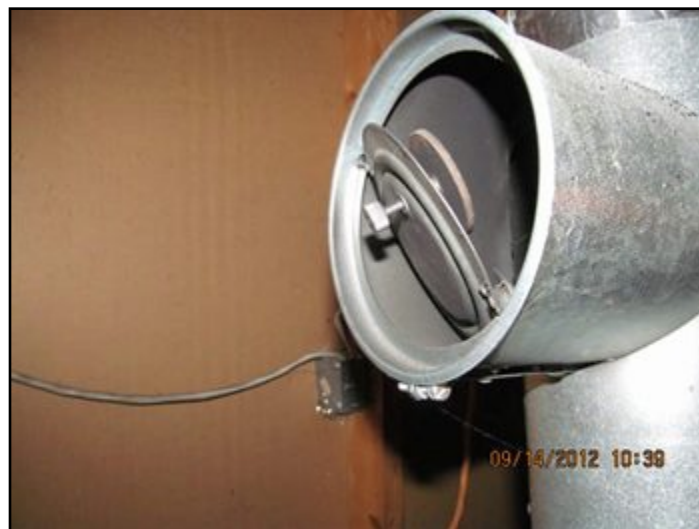
Barometric damper not working
