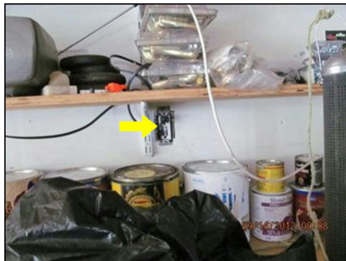
Damaged outlet
