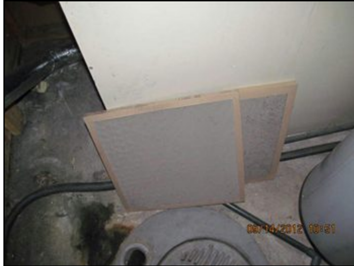
Furnace air filters removed
