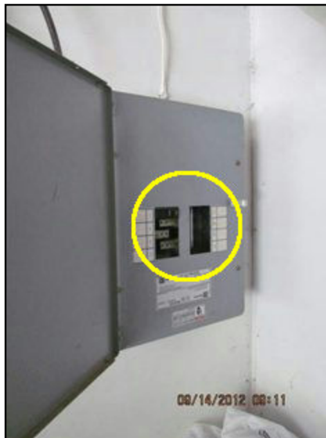
Openings in electrical panel
