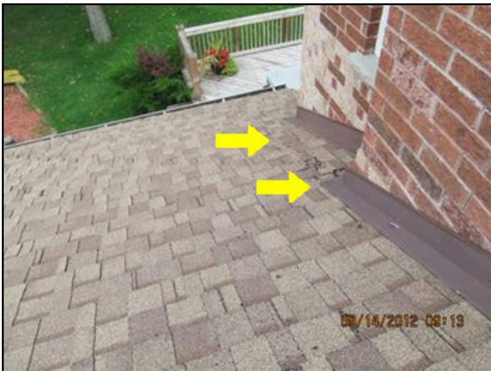
Shingles showing wear
