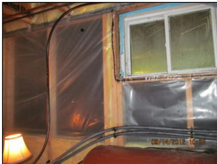
Missing insulation
