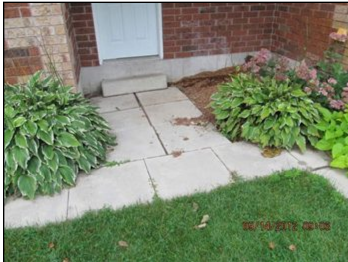
Walkway sloped towards foundation
