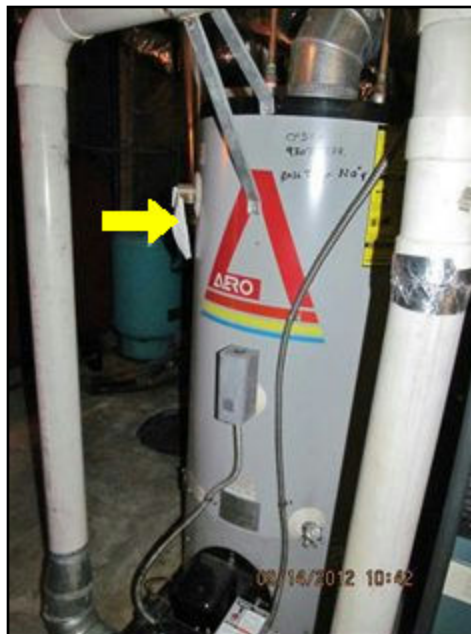
Discharge tube missing
