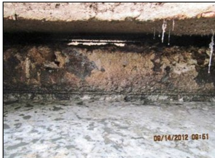
Interior baffle showing deterioration
