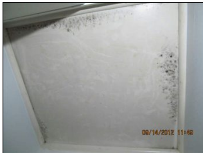
Air leakage around attic hatch
