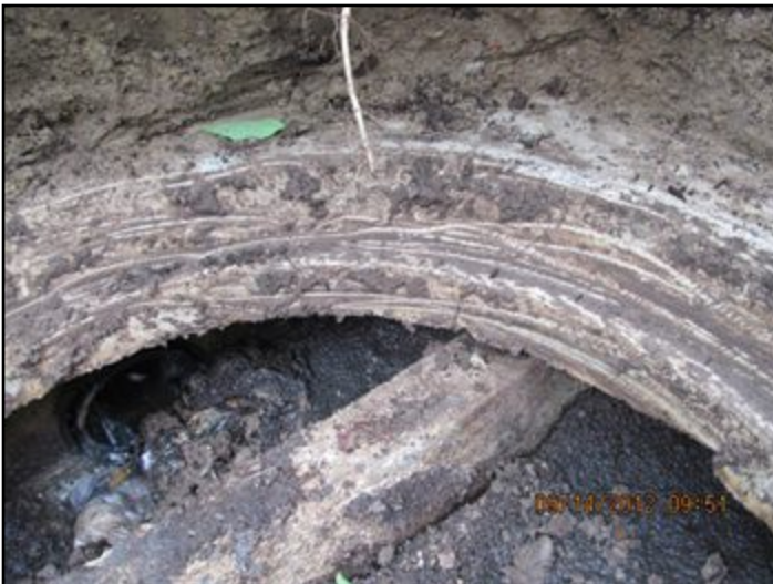
Cracks in septic tank
