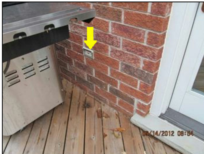
Weatherproof cover plate missing
