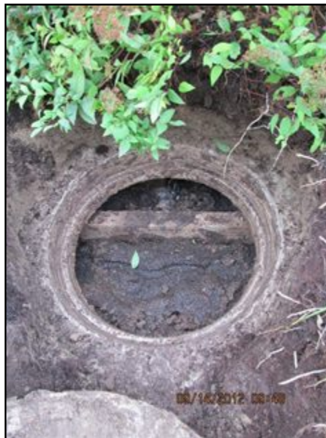
View of inlet chamber
