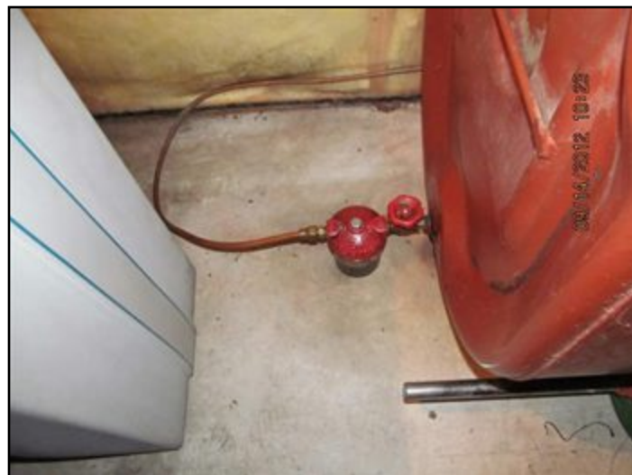
Location of oil tank oil filter
