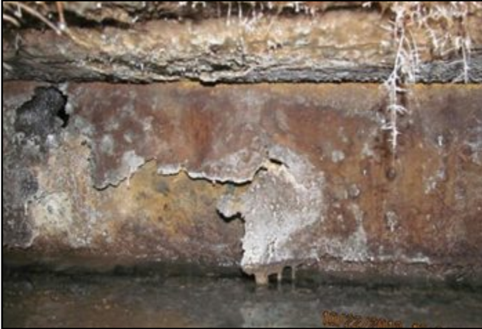
Outlet chamber showing deterioration
