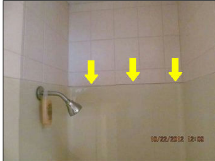
Cracking above shower panel
