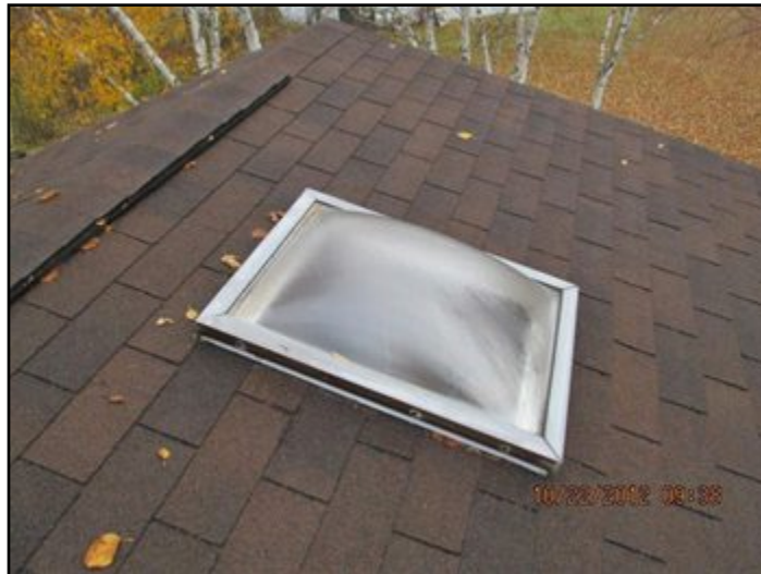
A lot of condensation on skylight
