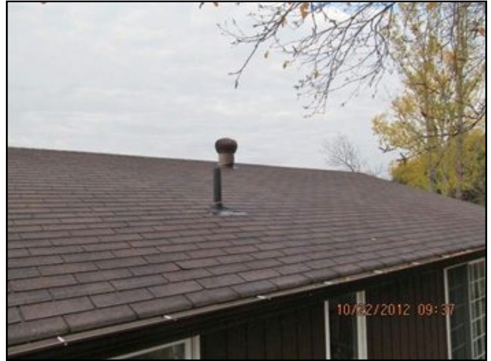
Wind turbine not enough ventilation
