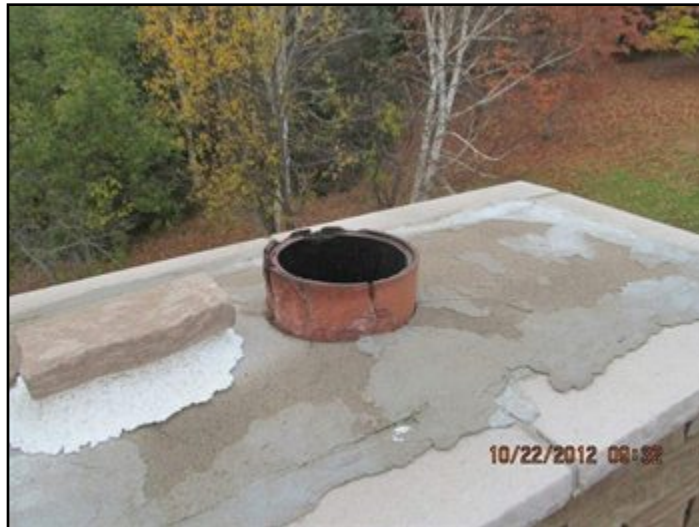
Top clay tile deteriorated
