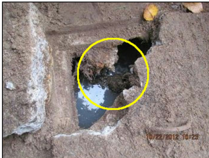
Outlet baffle just about gone
