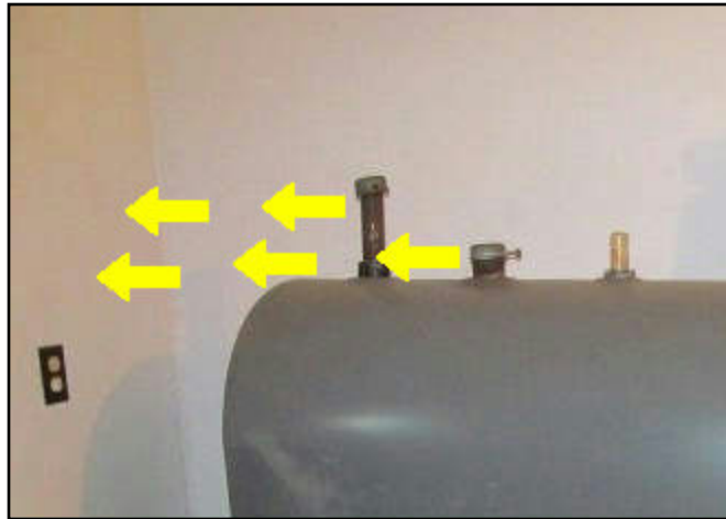
Oil fill/vent pipes in garage
