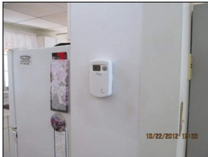
Existing oil furnace thermostat
