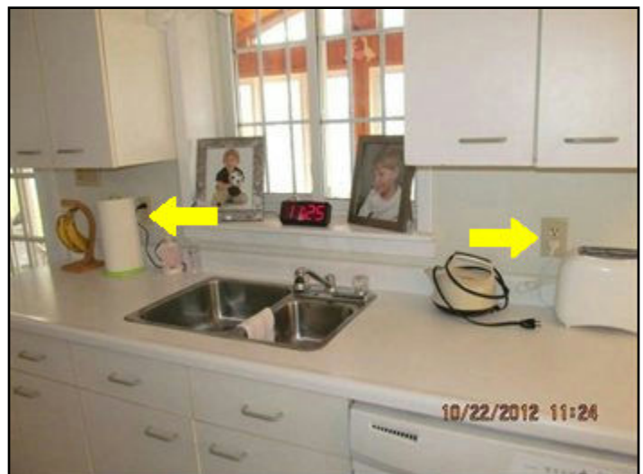
Recommend GFI protected outlets here
