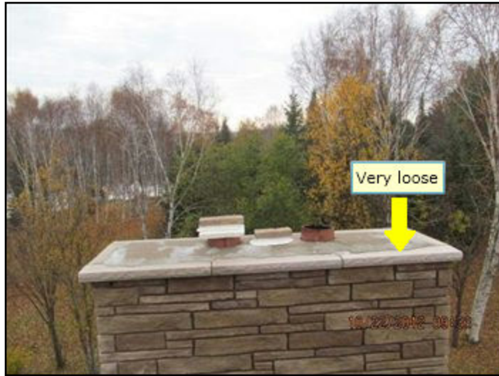
Chimney cap cracked
