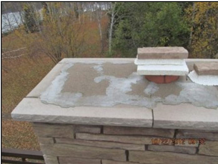
Chimney cap cracked
