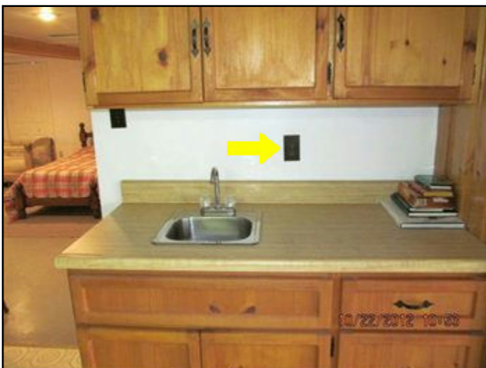
Recommend GFI protected outlet here
