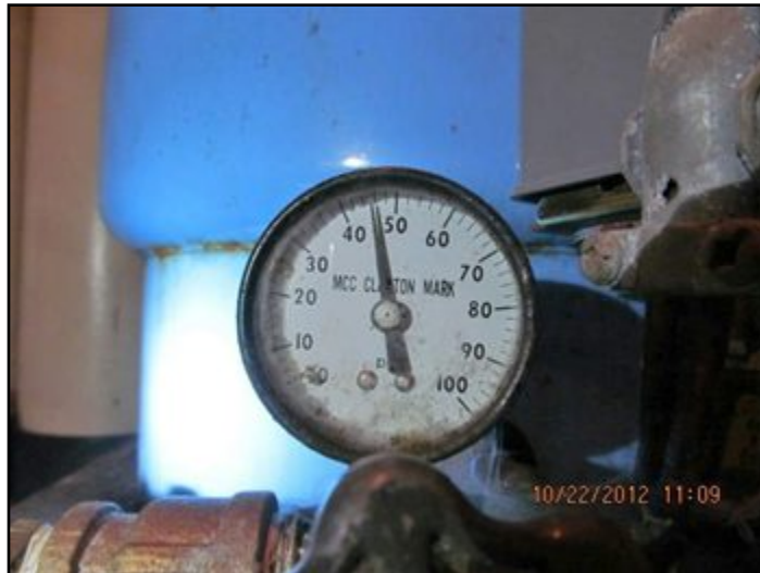
Water pressure at time of inspection
