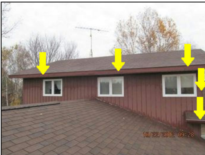
Missing gutter & downspout at rear
