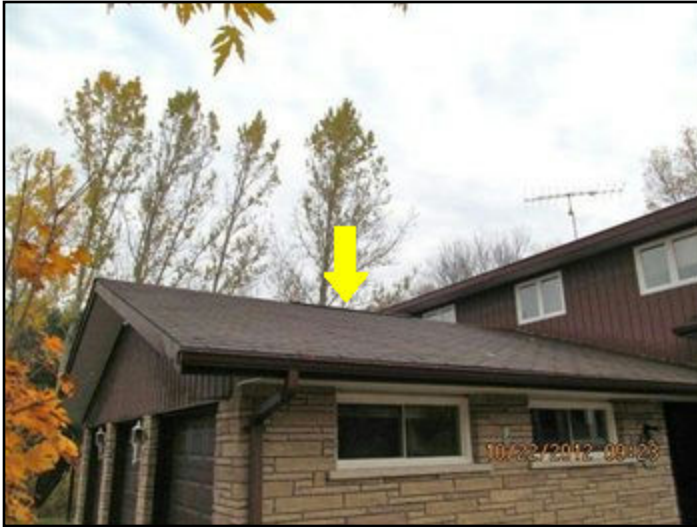
Not large enough ridge vent on garage
