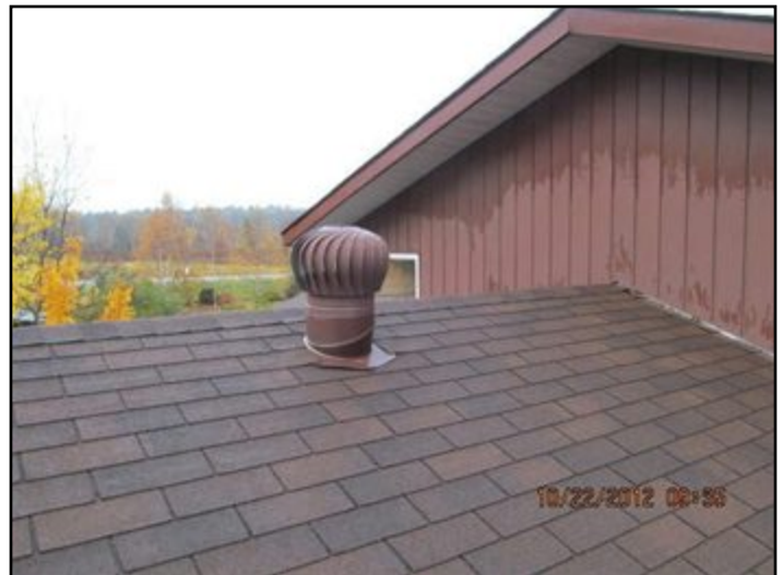
Wind turbine not enough ventilation
