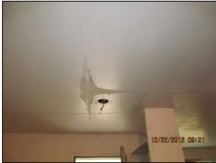
Previous water damage
