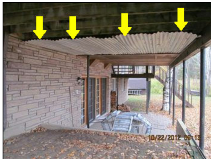
Plexi draining over wall
