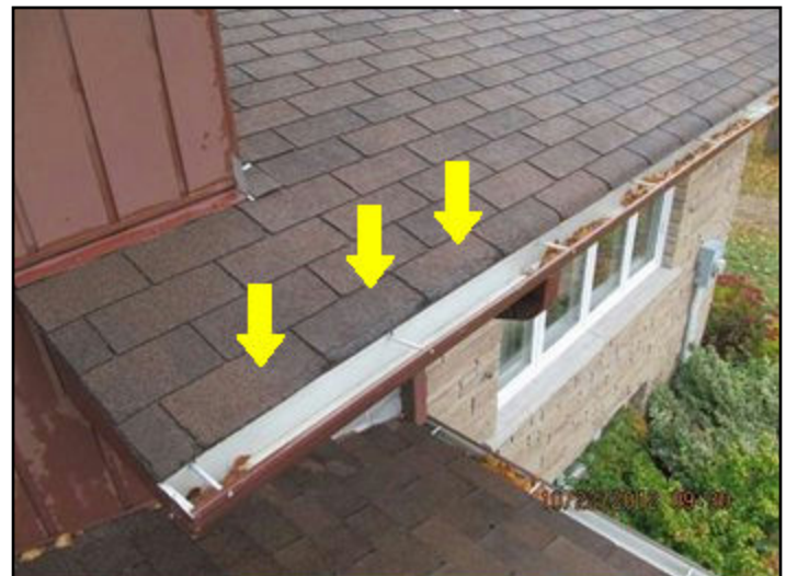
Shingles deteriorated
