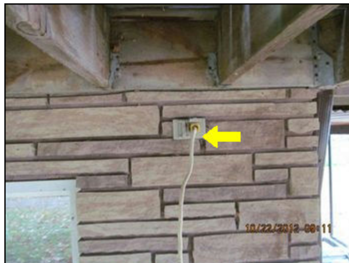
Permanent wire used as extension cord
