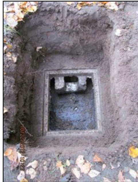
View of inlet chamber
