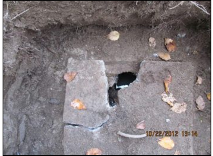
Outlet chamber lid badly cracked
