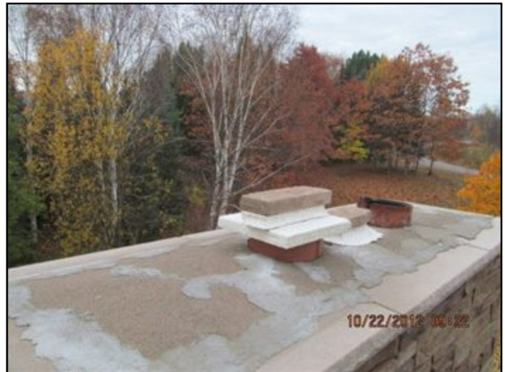
Chimney cap cracked
