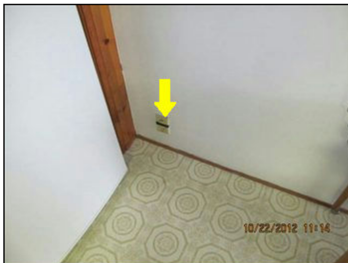
Central vac outlet closed off
