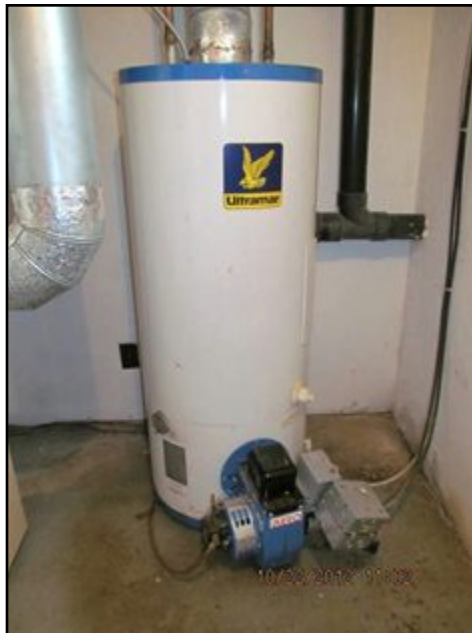
Oil fired hot water tank
