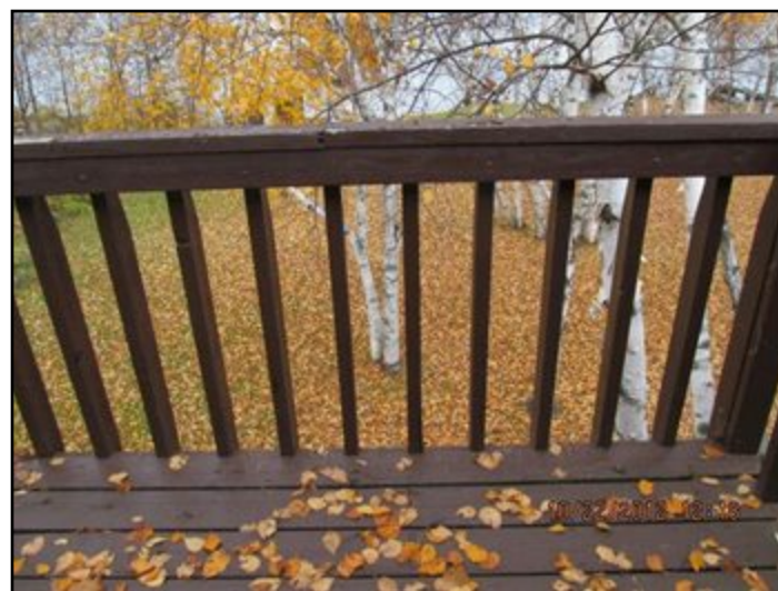
Spindles spaced too far apart
